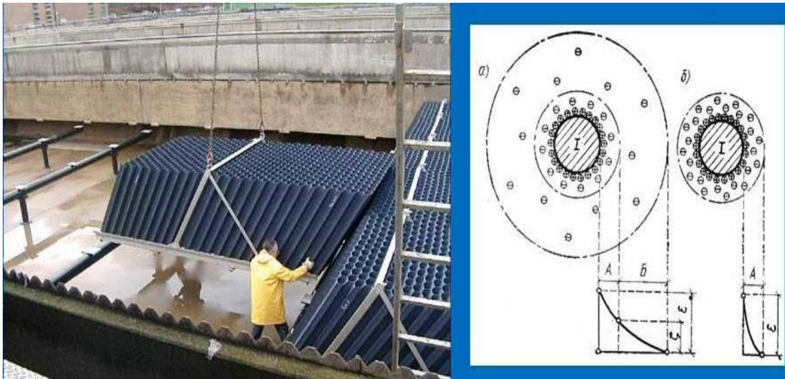
Picture 12 Water flocculation
